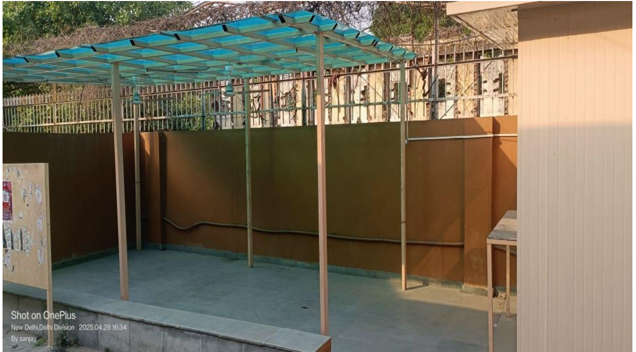
Exterior Repair Work
