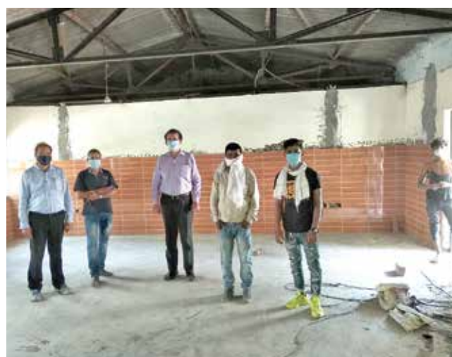
Kitchen construction work for School of Vocational Studies at Karampura Campus
