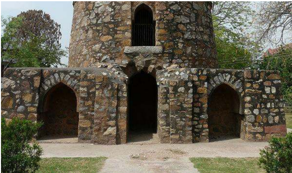
Chor Minar: Random Rubble masonry and arches (Credit: Ravina)
