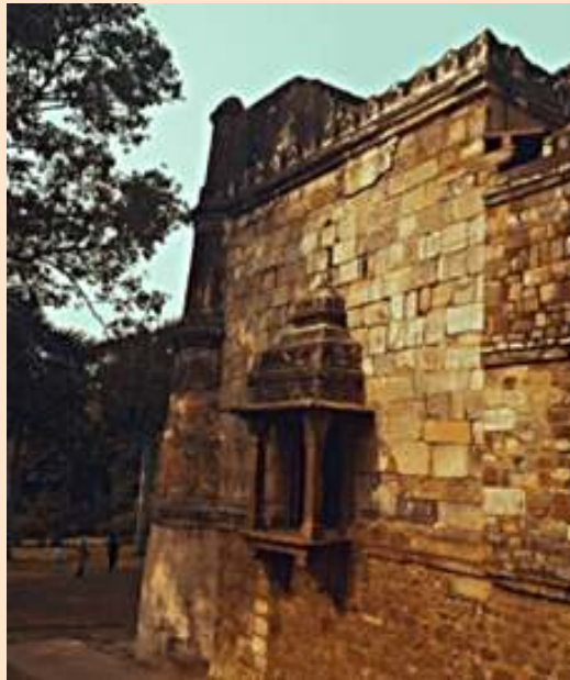
Fig 8 Source: Author, a Frontal structure on the Southern wall of the Mosque (view from the Western gateway of the Bada Gumbad)
